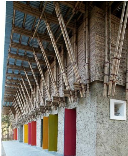
Figura 16: Exemplo de técnica Taipa-de-Mao. Handmade School – Rudrapur, Bangladesh. Fonte:< http://www.archdaily.com/51664/handmade-school-anna-heringer-eike-ros wag > Acesso em: 02/11/2015.
