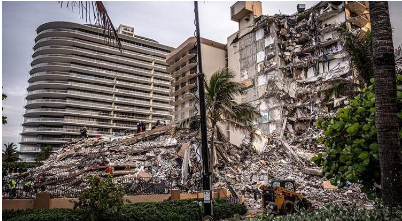
Figura 1 – Colapso do condomínio Champlain Tower South.
